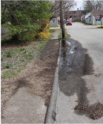
Poor drainage along Maple Street
