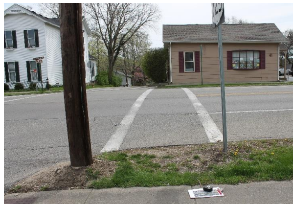
Crosswalk lacking signage and a curb ramp at West and Franklin
